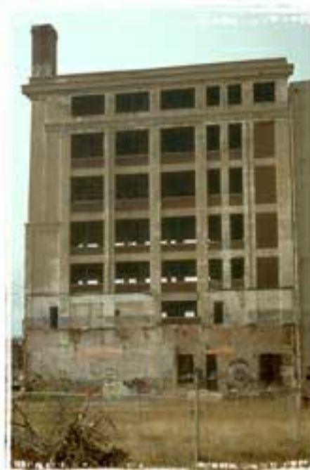
A long-vacant flour mill under renovation to lofts in the Central Platte Valley
