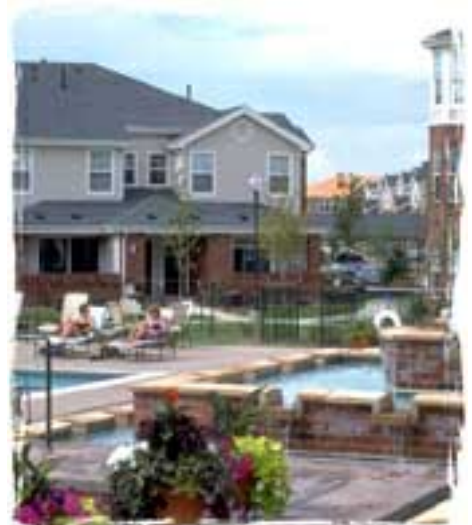
New rental homes at Lowry offer tenants attractive amenities
