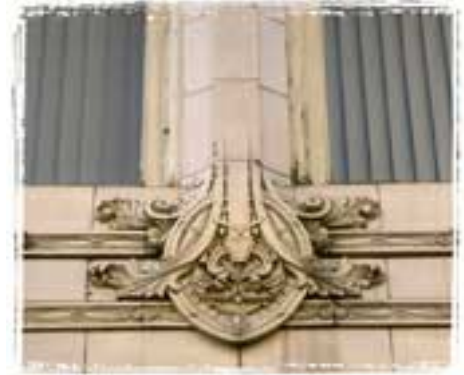
Beautiful terra-cotta detailing from a historic Downtown building
