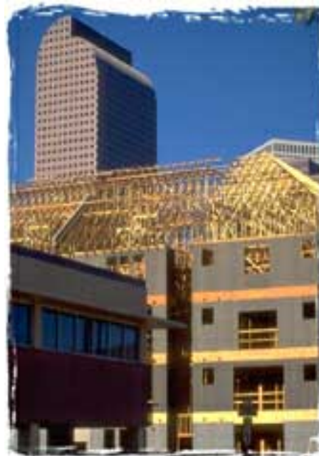
Downtown has experienced dramatic increases in new housing development
