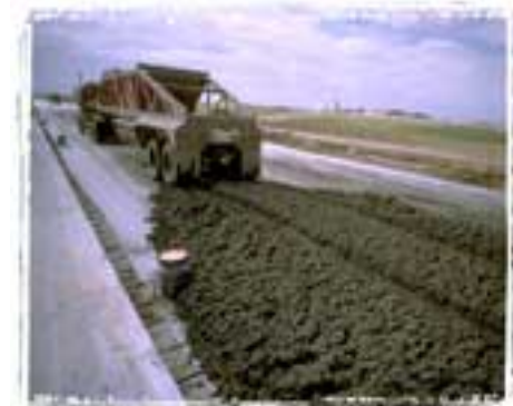
Roadway construction to support growth
